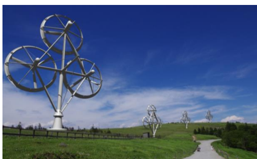
Fig.10 MRS on plains and hilly terrains (1MW MRS composed of 3 units of 300kW lens turbines)
