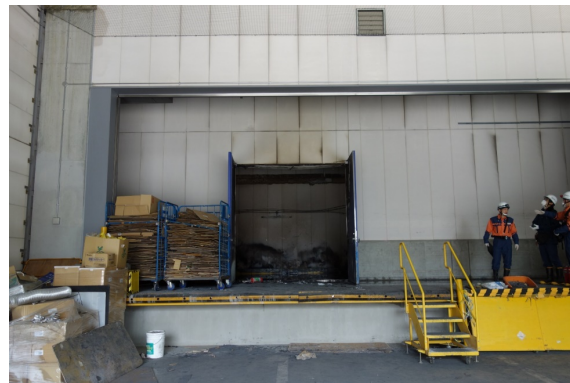
Fig. 5 Around the doorway of the used paper storage room.
