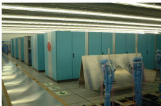
Fig.8 Installation of IN cabinets in the end of Oct. 2001.
