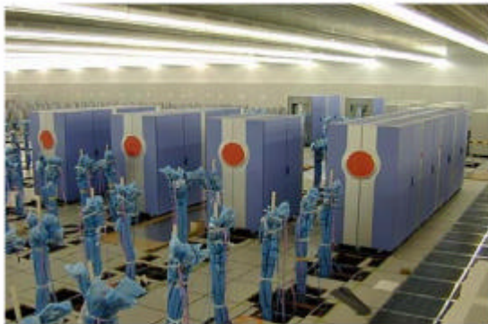
Fig.7 Installation of PN cabinets in Sept. 2001.
